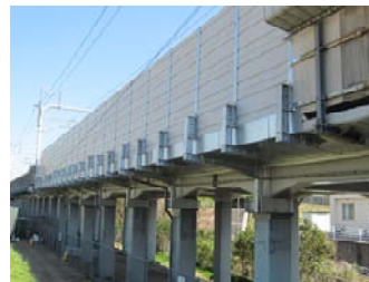
Fig.3 a completed noise barrier
