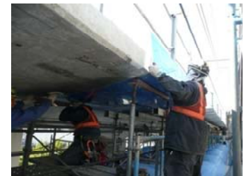
Fig.4 installed condition of steel plate
