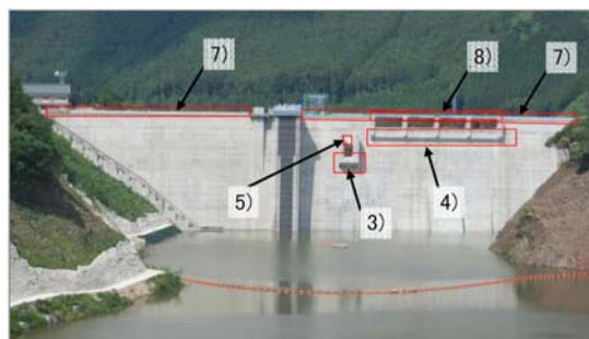
Photo-2 Precast concrete adoption part in the upstream side
