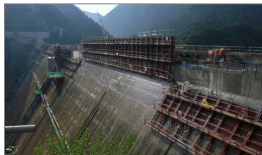
Photo-3 Precast concrete adoption part in the downstream side
