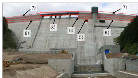
Photo-1 Precast concrete adoption part in the downstream side
