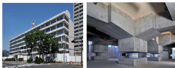
Photo.1 Exterior View and Finished Beams
