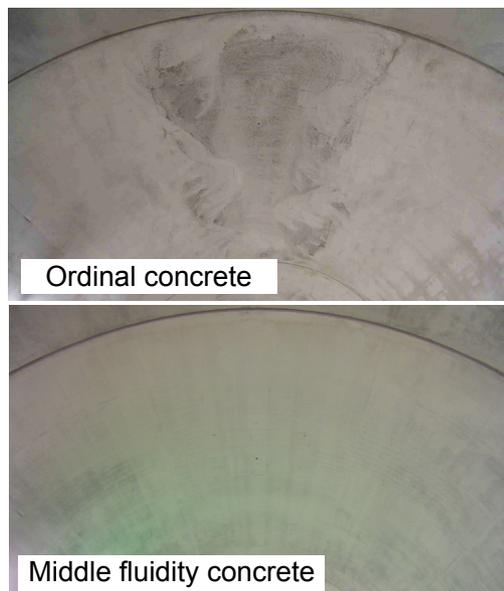
Photo 2 Surface of tunnel lining using ordinal and Middle fluidity concrete
