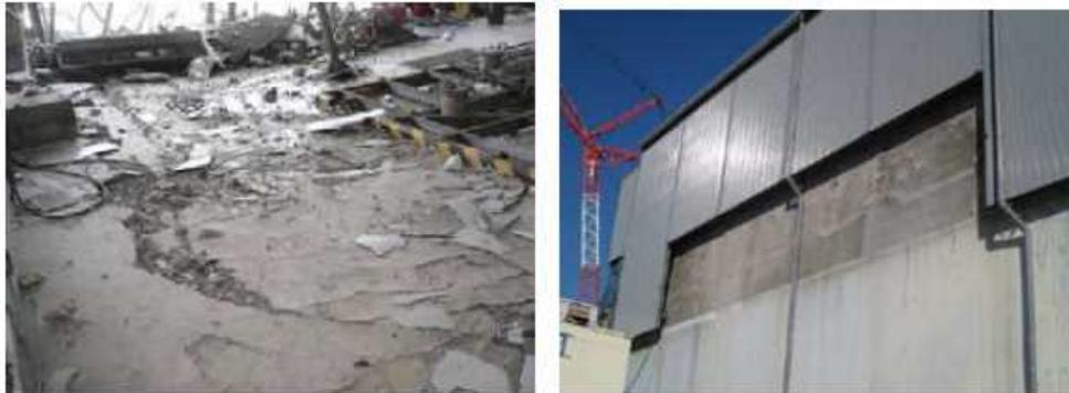
**Photo 2.1: Damage to Unit 4 (left) and Unit 4 after its repair (right)**
