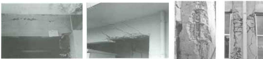
**Photo 1: Examples of bond splitting fractures**
