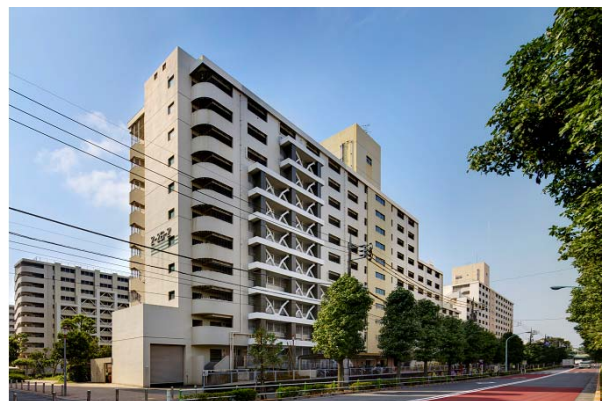
Photo 1. View of the building after reinforcement
