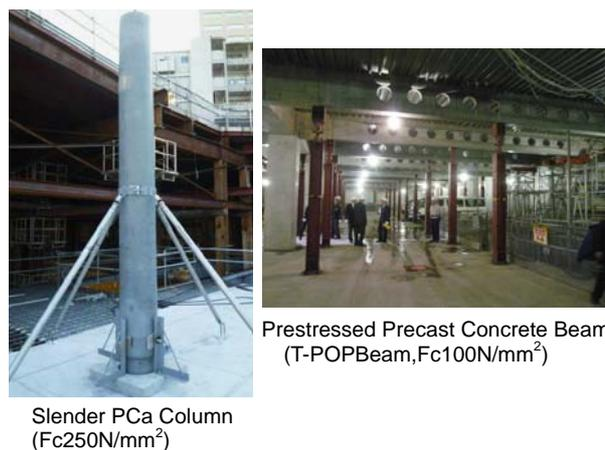
Fig.3 Allocation of Slender PCa Column and Prestressed Precast Concrete Beam
