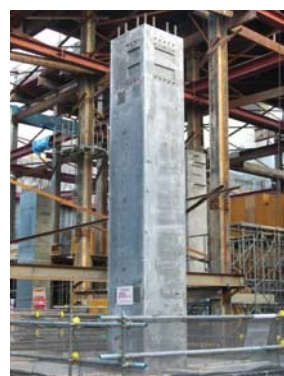
Photo 3 Erection of precast column
