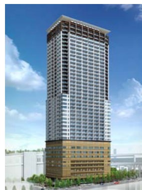
Photo 1 The superhigh-rise condominium in which precast concrete with 200 MPa was used
