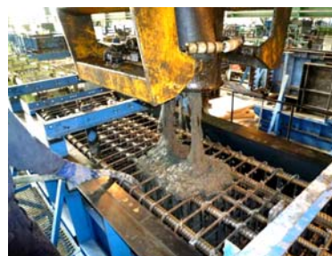
Photo 2 Concrete placing in horizontal position
