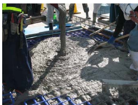
Photo.2 Placing of FRCC
