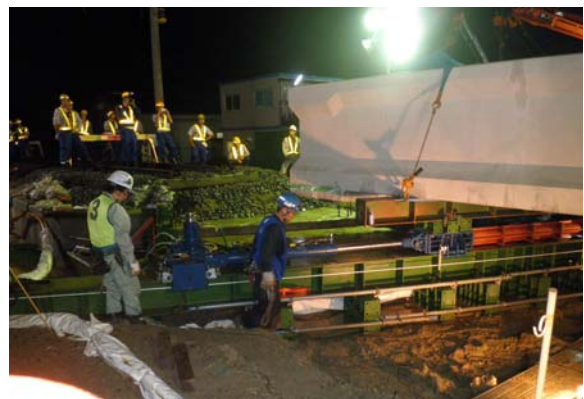
Photo 2 State of erection of UFC girder
