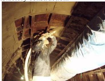
Photo.1 Spraying of filling mortar
