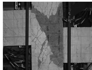
Fig.3 crack pattern at final stage in specimen with the distance of a half beam depth
