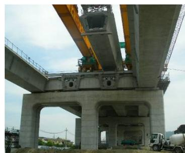
Photo.4 Erection of the girder
