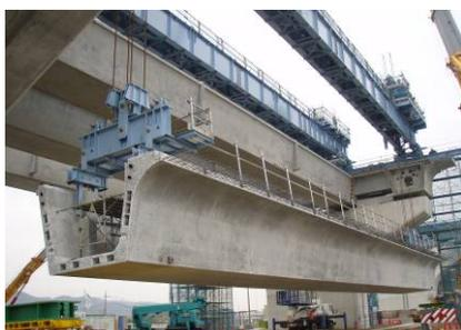
Photo.2 Erection of the U-girder
