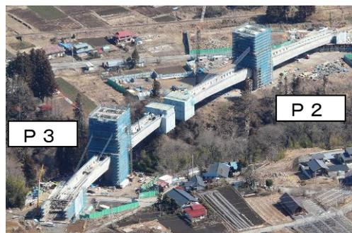
Photo 1 Cantilever erection in progress
